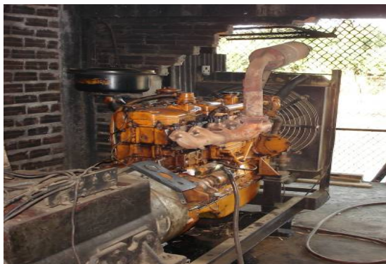
Figure 4: Village grid generator for 250 households, Cambodia
