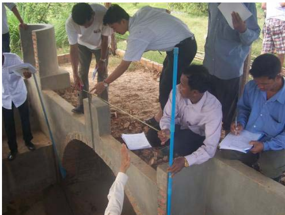
Figure 26: Course 7, Practiced with standard plan measurement to the demo bio-gas plant
