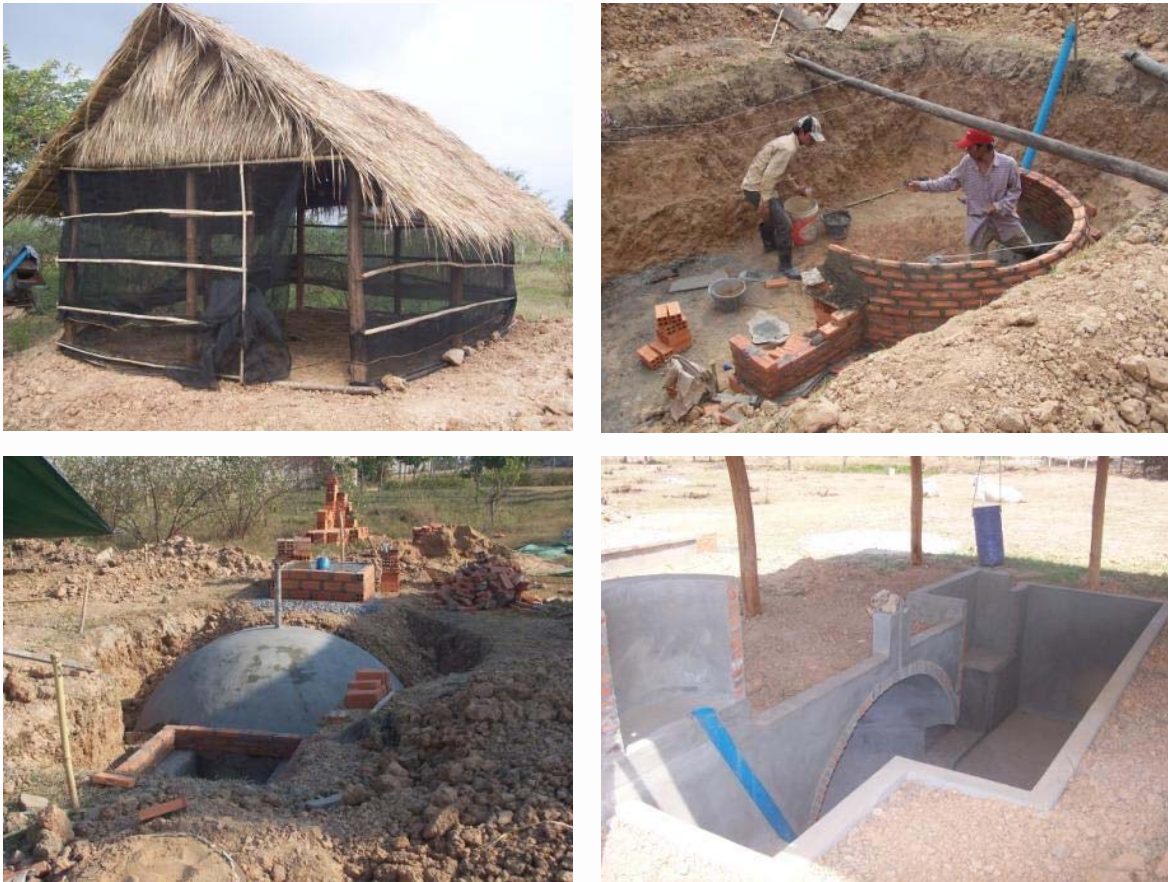
Figure 56: Construction of biodigester plant and cross section at the COMPED training centre
