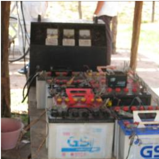
Figure 51: Charge controller and Batteries
