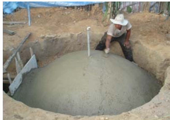
Figure 36: Biogas plant building
