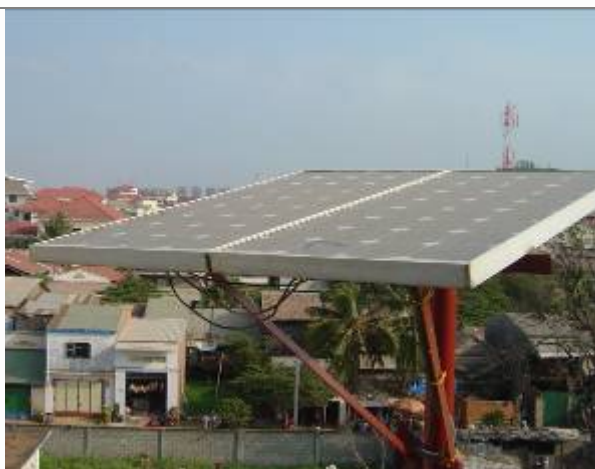
Figure 58: Solar panel with a capacity of 150Wp (each panel 75Wp)
