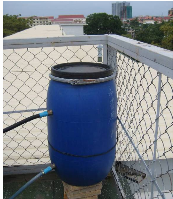
Figure 65: The storage tank with a capacity of 150L
