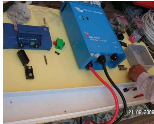
Figure 38: Installation of inverter and charge controller
