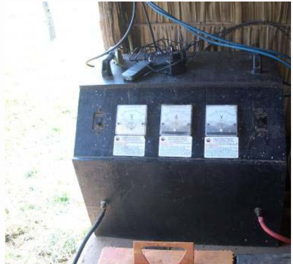
Figure 50: Charge controller
